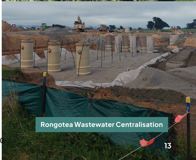
Rongotea Wastewater Centralisation
