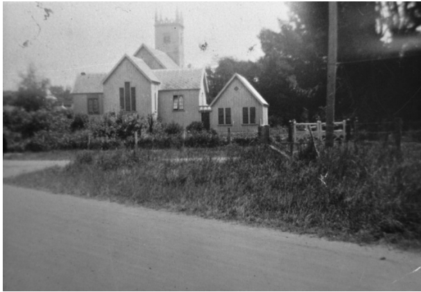
Figure 1 St. John's Church showing the attached Sunday School at right that was built in 1885 and burnt down in 1909. (Source: Feilding Library, ID: CHS:ce1: http://feilding.recollect.co.nz/nodes/view/17573 )
