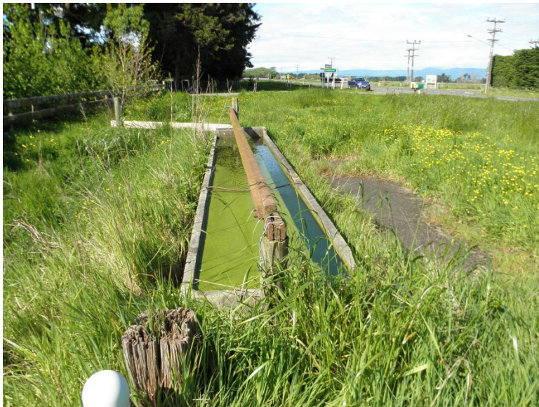
Figure 3 The trough with its concrete foot pad in the foreground. The rail along the length of the trough was to reduce the temptation of livestock to jump into or over the trough, and also to make it easier for stock to drink from both sides of the trough without interfering with each other. Looking in the direction of Cheltenham and the Colyton Road intersection - 27 November 2016
