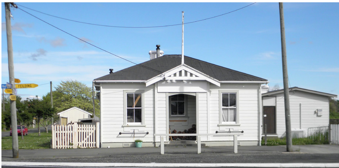
The former Halcombe Post Office (23 October 2016; Photo: Val Burr)
