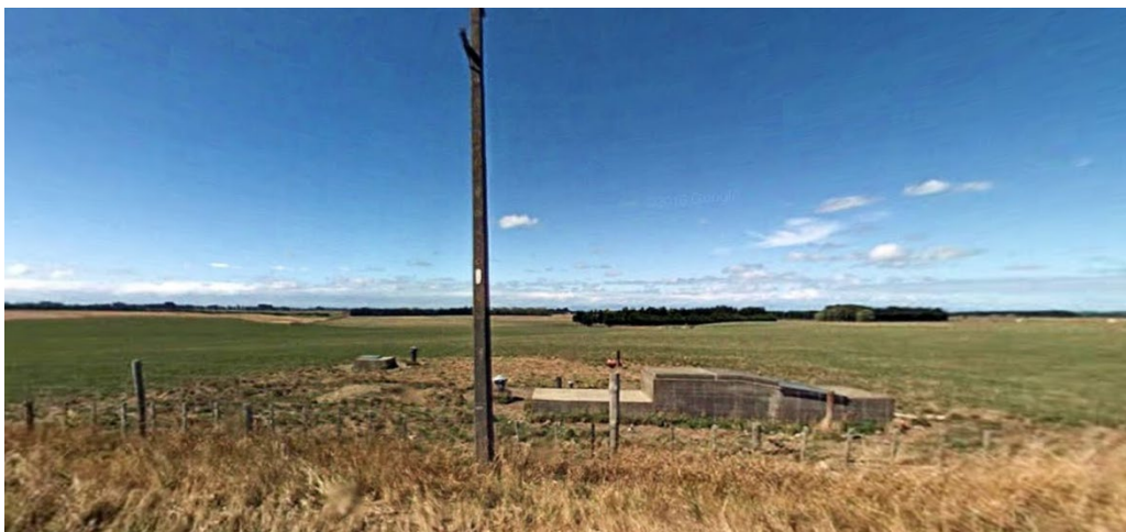
Figure 3 The Ohakea Operations Room still underground, as photographed by Google Street View in March 2008, before the soil was removed from the top of the concrete room. The soil had been cleared by February 2010 (Google Street View image).
