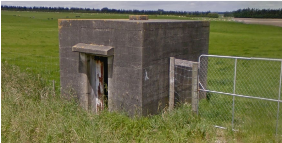
Figure 4 The small structure that contained the engine that powered the operations room (Source: Google Street View, November 2013)
