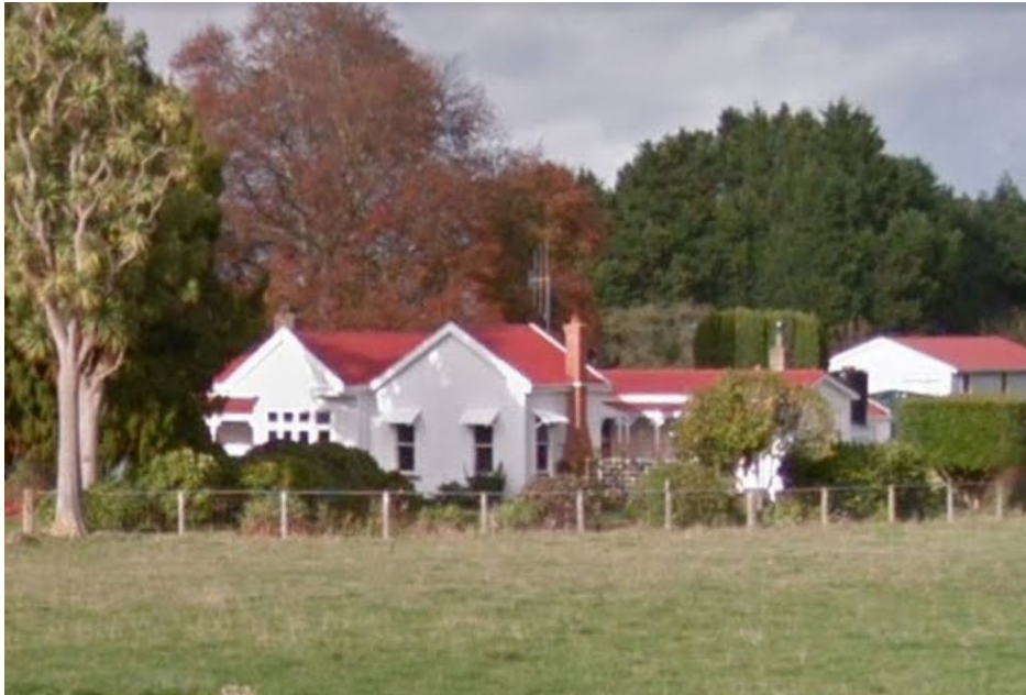
291 Haynes Line. This photo shows the comparatively low-roofed extension at the back of the house that was added in 1964, as shown on the property's Building Permit plan. (Source: Google 'Street View', May 2015)
